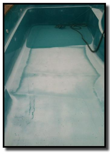
If the gelcoat has severe damage by the salt (calcium chloride) and it is visible when hydrated then the solution is to remove the salt from the surface of the pool. To date we have not been able to identify a chemical solution for the salt removal. As a result, the surface needs to be buffed and polished to firstly remove the salt build up and then to restore the luster of the pool surface. It is however very important that you speak with your builder before draining the pool.
